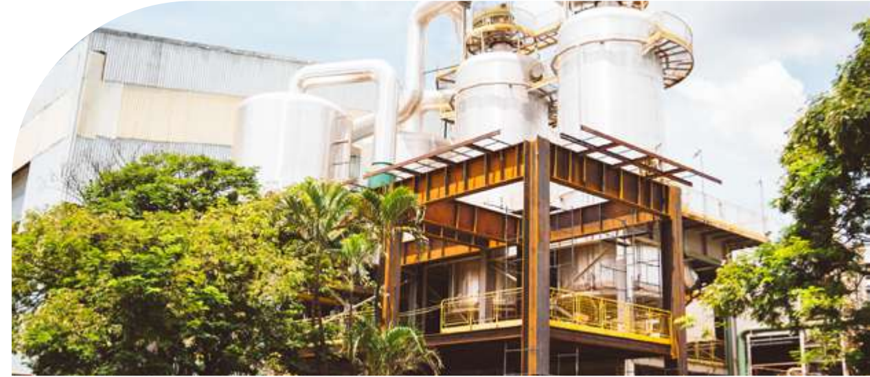
Vacuum pan and pre-evaporators, and, at the front, structure for new evaporators and vacuum pans for the 24/25 crop (Sugar Plant)
